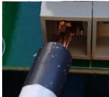
Poor termination
